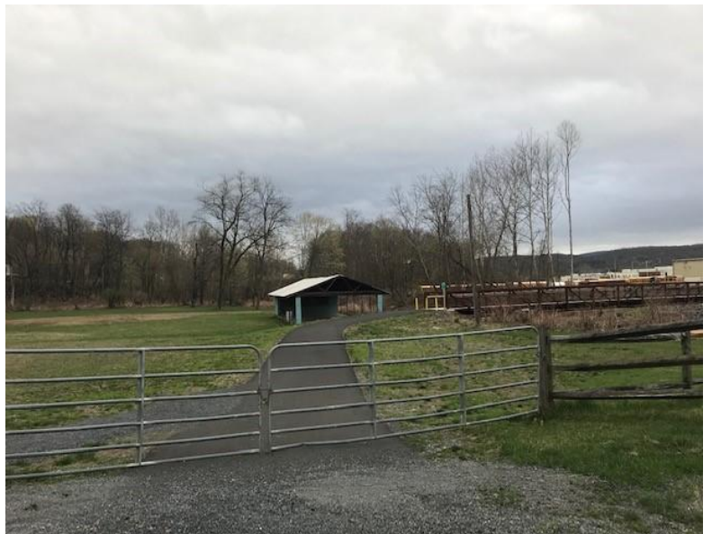
Existing Path to Pedestrian Bridge
